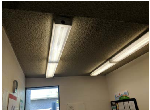
No damage ceiling in office 3
