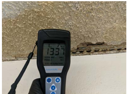
RLU for work area
